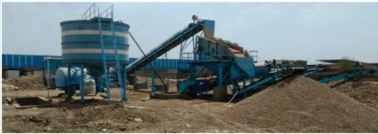
Various components and instruments at C&D waste management plant. Photo credits: Saxena et al. 2018.
