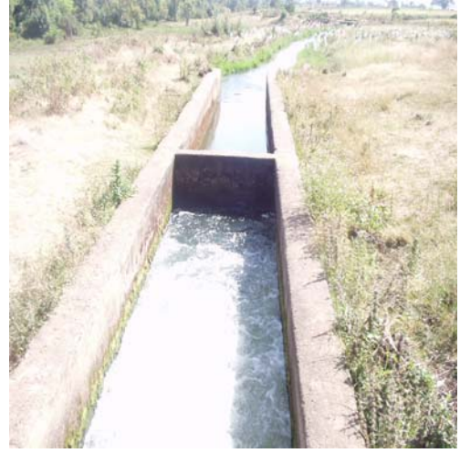
Plate 4.3 Main Canal partly lined
