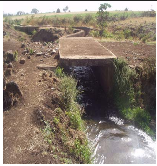
Plate 4.3 Main Canal partly lined
