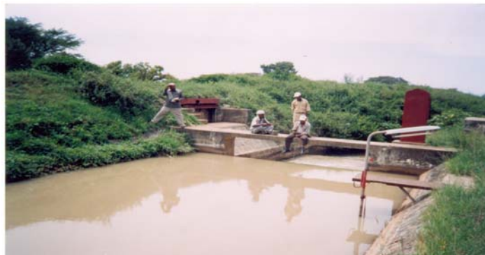
Measuring discharge from cippoleti weir at Wonji
