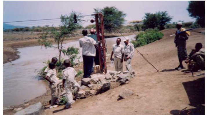
Preparation for work at Nuraera
