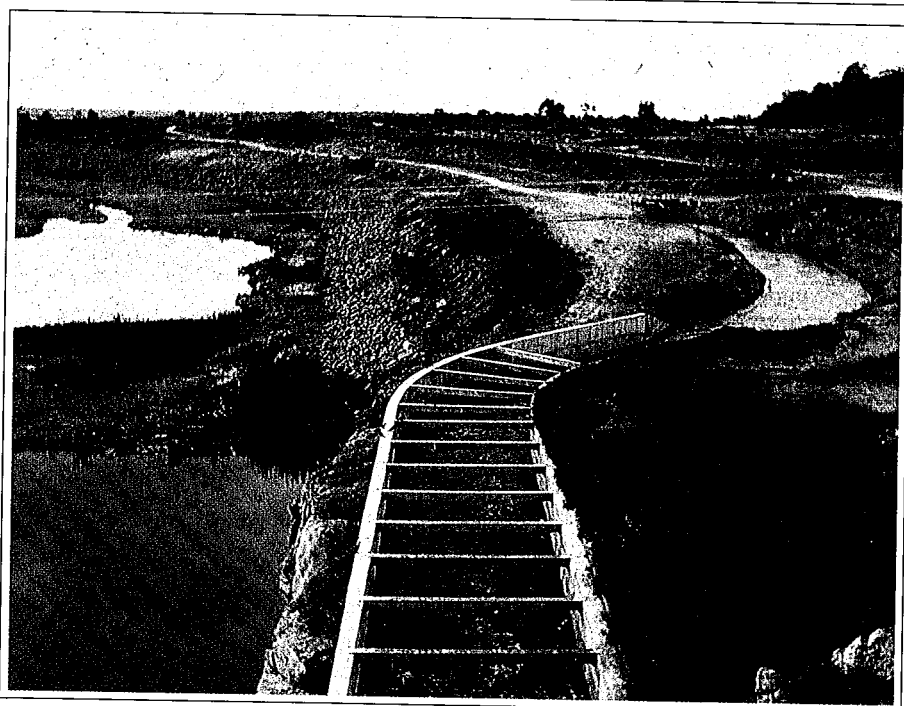
System rehabilitation is gaining popularity over new construction.
