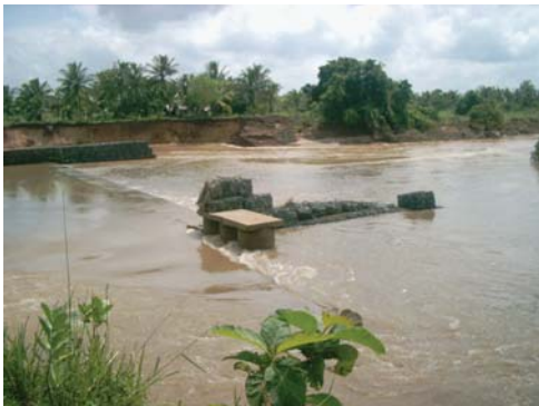
Damages caused by flood water at the Deduru Oya dam close to Puliyankulama.
