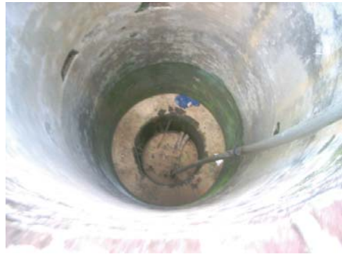
Aspect of the dried well and dropped tubewell instrument to the bottom.
