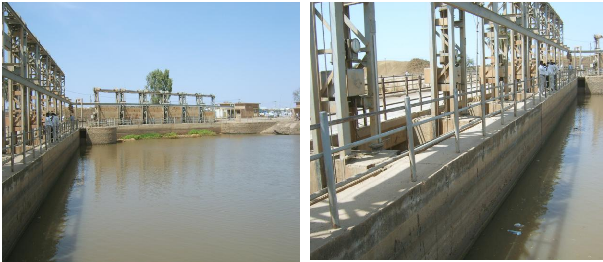
Figure 2: Regulators at Abu Rakhm Barrage
