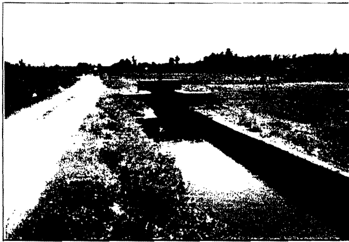
A 390 m section of the main canal in the head reach has underground construction.
