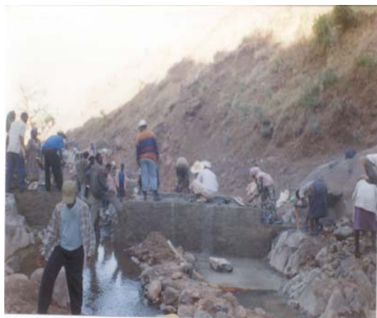
Figure 2. Construction of diversion weir and main canal at Harbu small-scale irrigation
