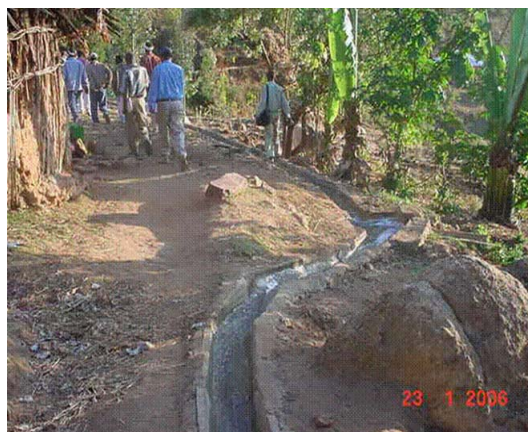
Figure 3. Canal reinforced by cemented wall to reduce water loss, at Metta woreda, East Haraghe Zone
