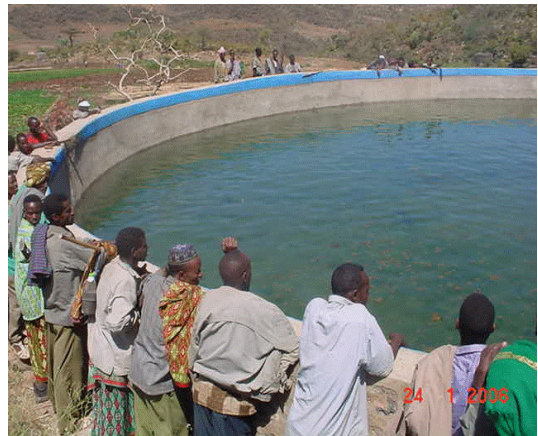
Figure 1. Water storage constructed at high elevation at Goro Gutu woreda, East Haraghe Zone
