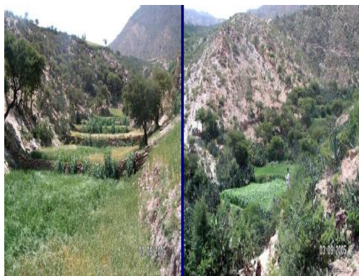
Figure 3. Traditional sediment storage dams
