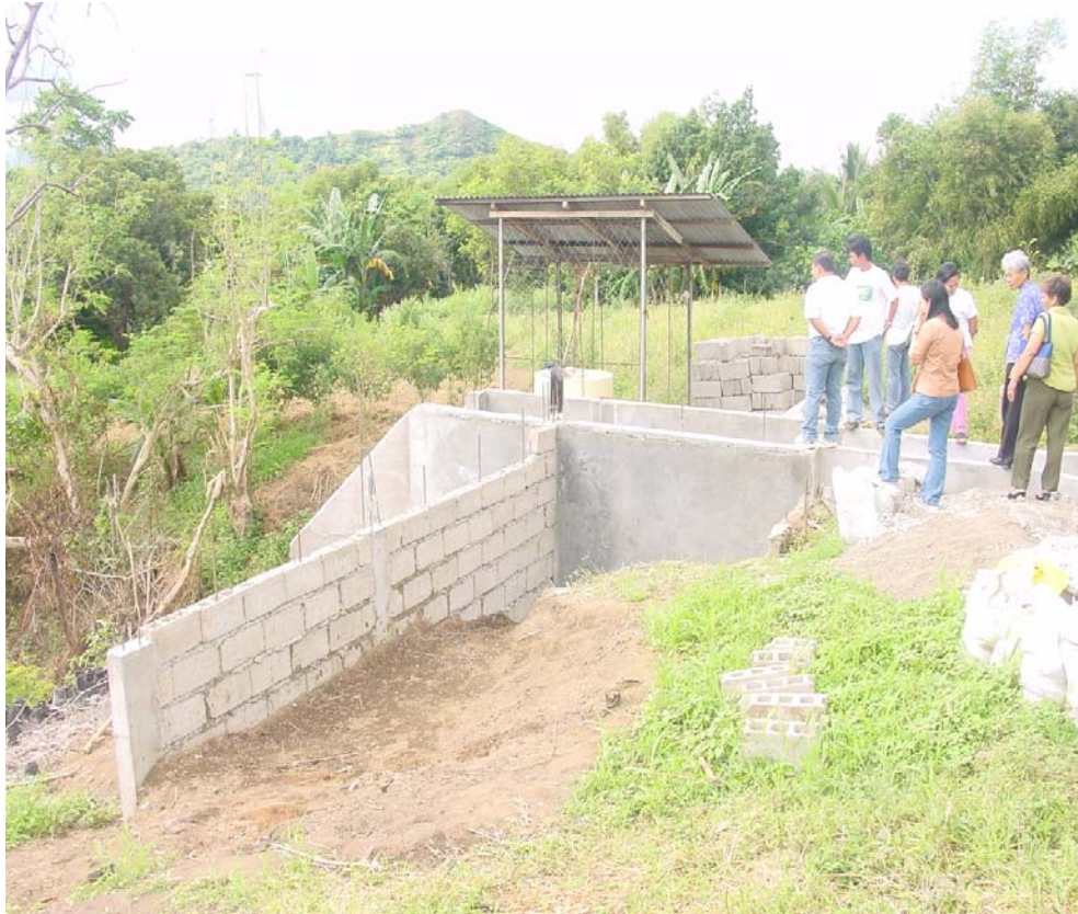
Figure 6. Weir at the Maria Paz site
