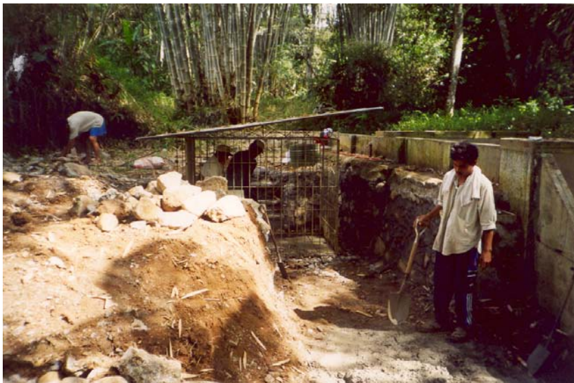
Figure 1. Repair and rehabilitation of the main weir
