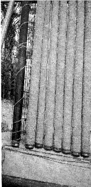
**Plate 2.** Jute and nylon-wir wrapped coir as strainer in single strainer skimming well.
