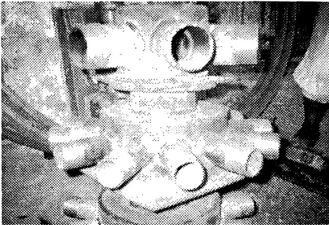
Plate 4. T-joint for connecting strainers to the pump.
