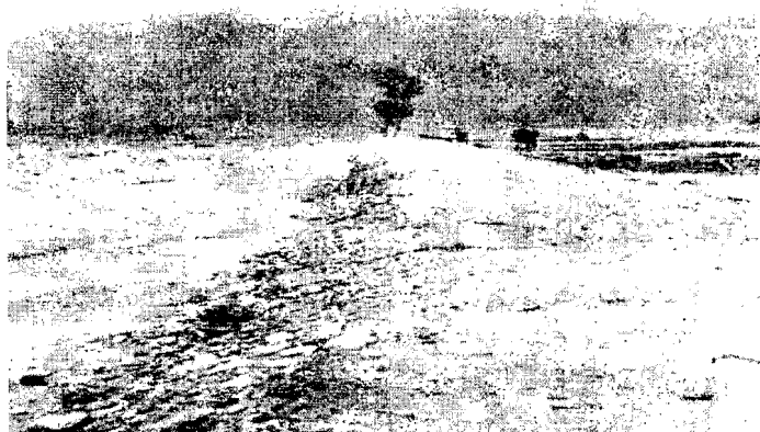
Photo 4a: Due to constrained waterway floodwater overtopped the right embankment. Spurs protected the embankment (Refer K1 )
