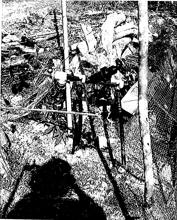
Figure 8.3.3. Pressure regulator valve and fertilizer injector.
