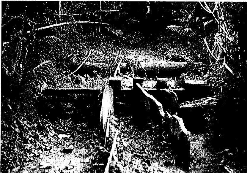
Figure 7.0.3. Drop built ahead of a proportioning weir to create a pool and reduce the approach velocity, Parbat, Nepal.
