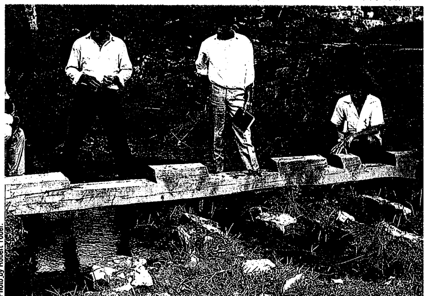
Figure 7.0.2. Water proportioning weir removed from operation during the dry season when water is more easily delivered by timed rotation among secondaries.
