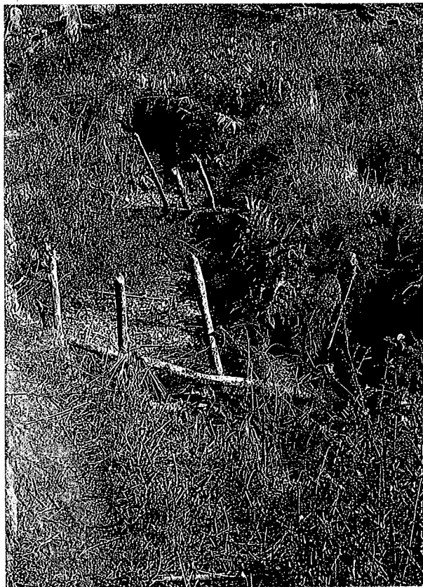
Figure 7.0.6. Farmer-built drop structure using forest products in Nawal Parasi, Nepal.
