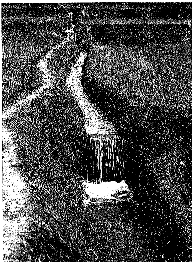
Figure 7.0.5. Farmer-built dry stone masonry drop structure in distribution canal in Gulmi, Nepal.
