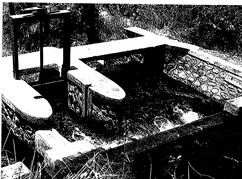
Figure 7.4.3. A traditional weir-type divisor made of concrete, which is a modification of a gated flow divisor built at the request of farmers.
