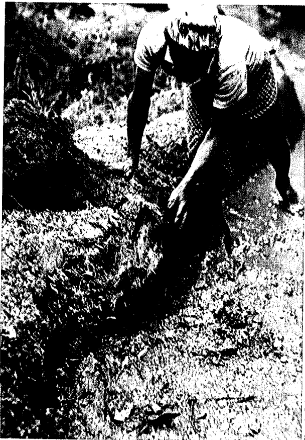
Figure 6.0.6. Red-clay lining applied by farmers as a temporary measure to reduce water losses from the canal during a critical water-shortage period.
