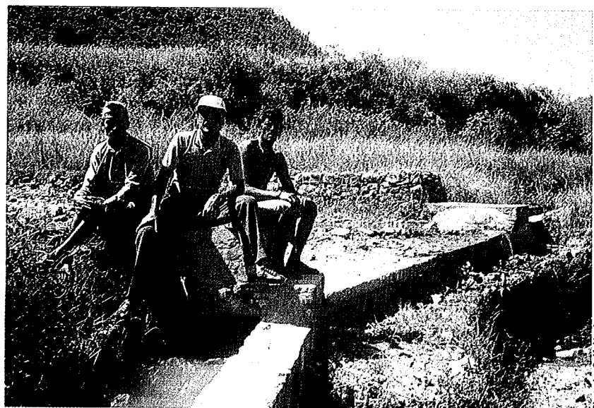
Figure 6.4.2. Completed superpassage in the Dhand Khola Irrigation System, Kabhrepalanchok District, Nepal.
