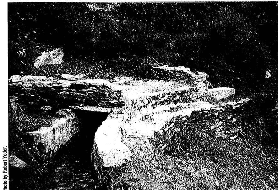
Figure 6.0.2. Superpassage in Nepal that should have been shifted several meters toward the hillside.
