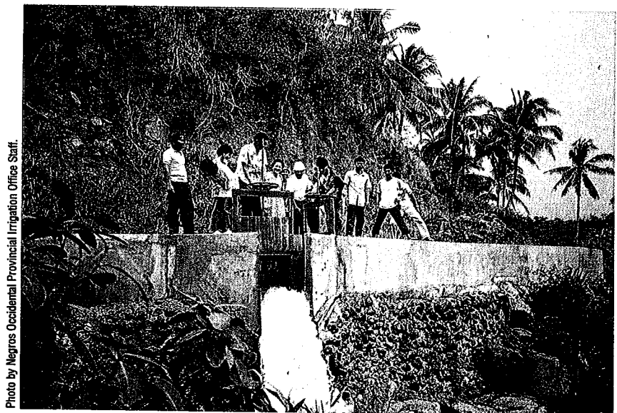
Figure 6.11.1. Sluice gate and inlet gate upstream of the bench flume in the Cabacungan Communal Irrigation System, the Philippines. The bench flume runs for 90 m to the right of the group of people.
