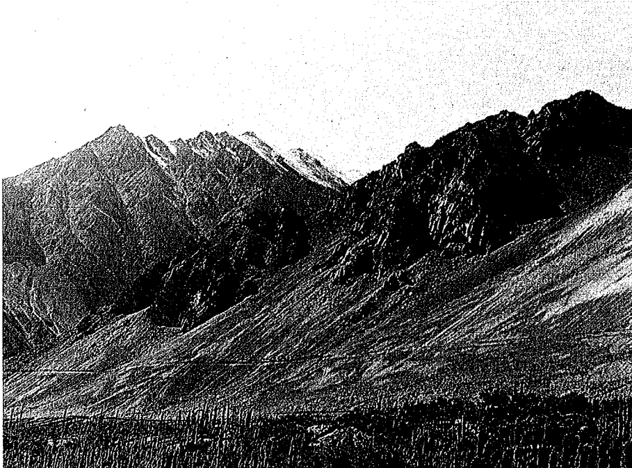
Figure 6.2.6. View of part of the previously developed command area with the channel visible as a line on the scree.
