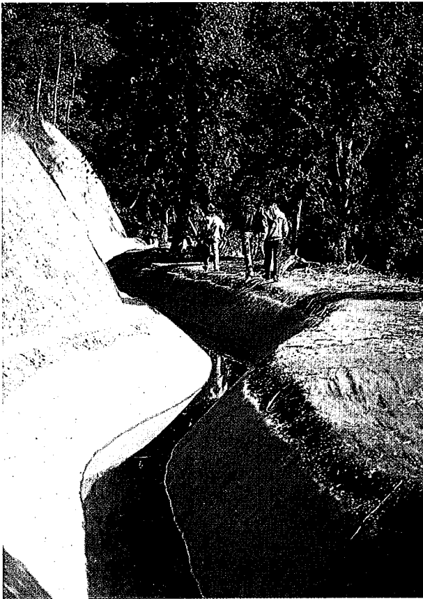
Figure 6.14.1 Soil-cement lined section of canal, Andhi Khola Project, Nepal.
