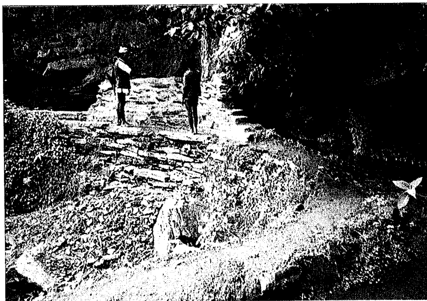
Figure 6.0.3. Superpassage in Nepal built against the hillslope.
