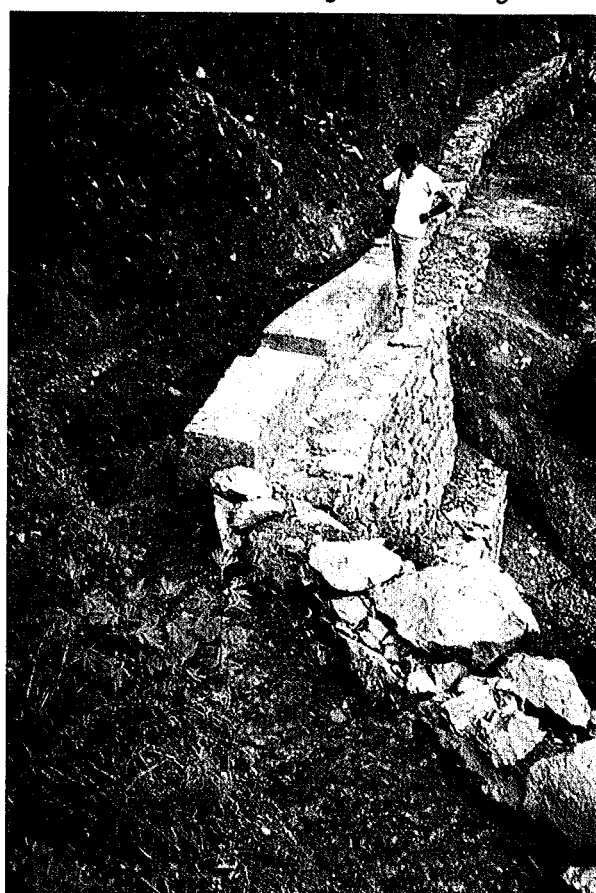
Figure 6.0.1. A level crossing in Nepal where the spillway crest is too high above the canal bed. The spillway should be wider and an orifice should be constructed to control drainage water entering the canal.
