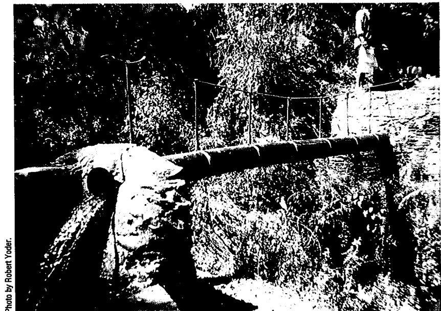
Figure 6.6.1. Suspended pipe aqueduct in Sindhupalchok, Nepal.
