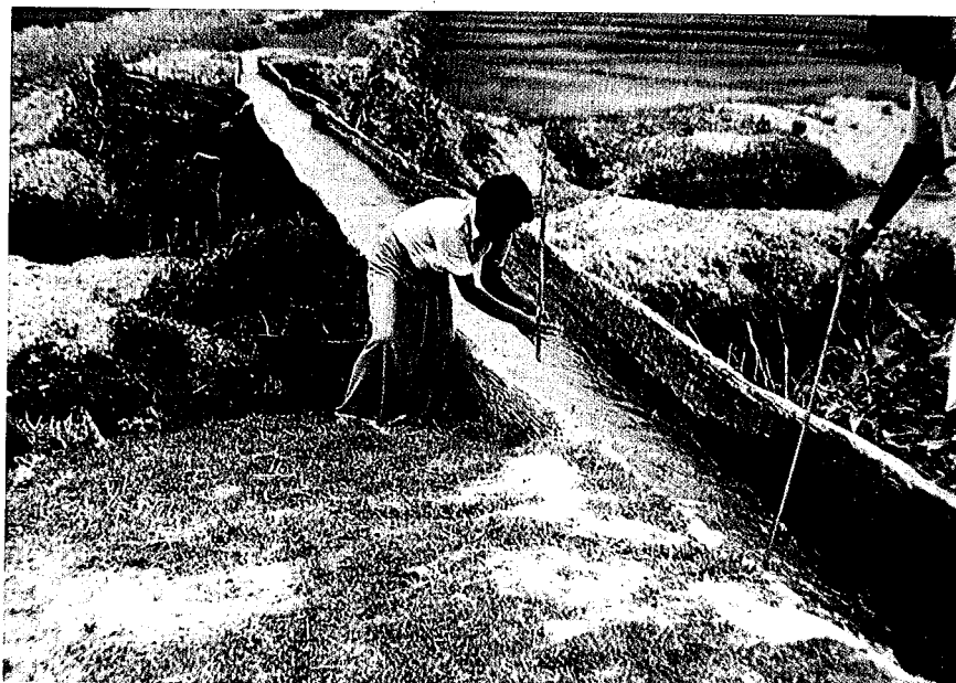
Figure 6.0.4. Hollow log used as an aqueduct in Nepal.
