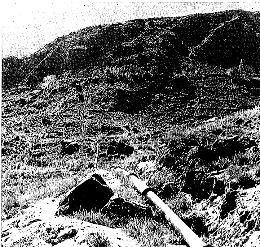
Figure 6.16.2. View, from near the inlet tank, of the siphon pipe crossing the valley, Chalt, northern Pakistan.
