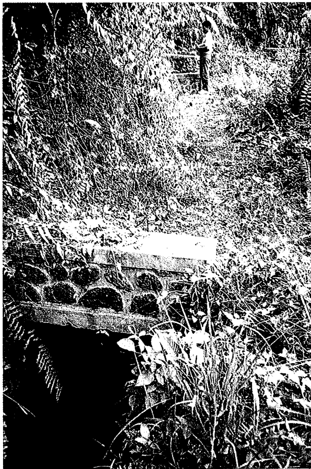
Figure 6.9.2. Concrete slabs used to cover masonry canal, Bali, Indonesia.
