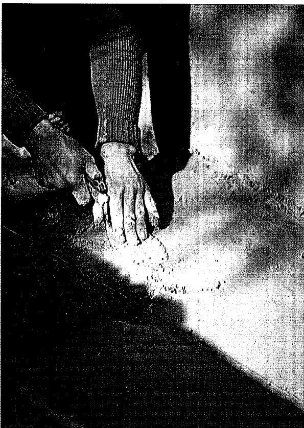
Figure 6.14.3. Soil-cement application for lining canal in Nepal.
