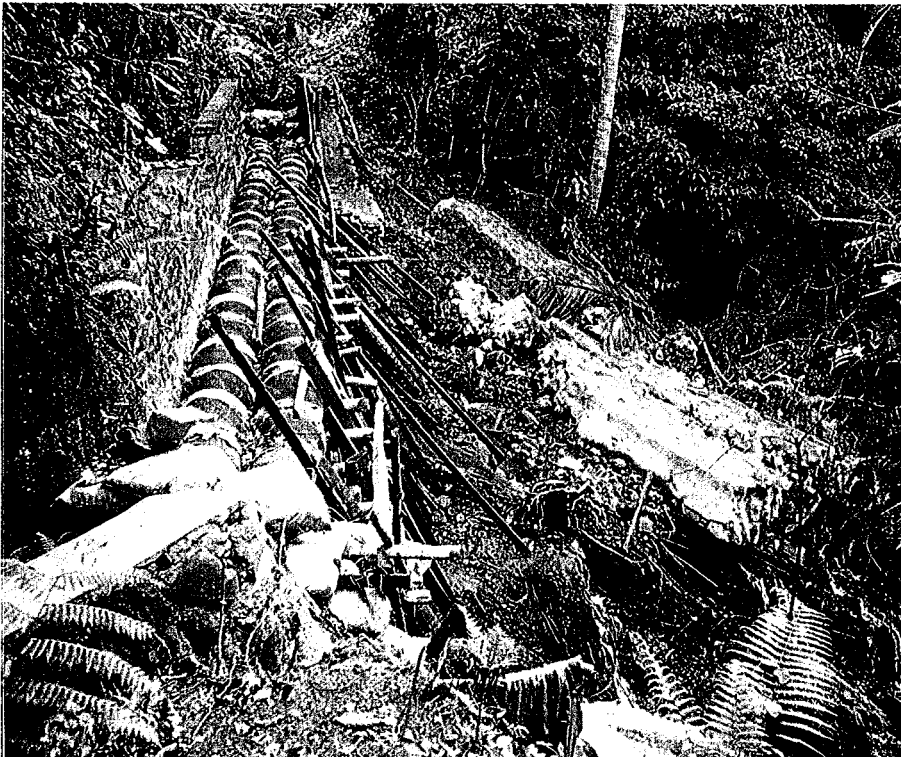
Figure 6.9.1. Pipes made from drums joined with bituminous-covered fabric which replaced a collapsed masonry wall, Bali, Indonesia.
