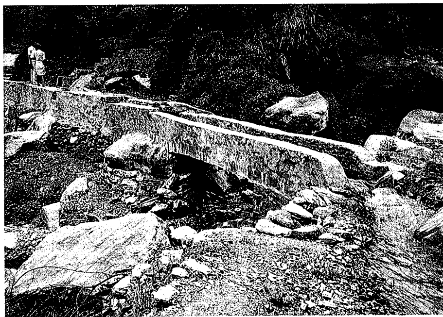
Figure 6.7.3. Reinforced concrete aqueduct with collapsible side walls, Sindhupalchok, Nepal.
