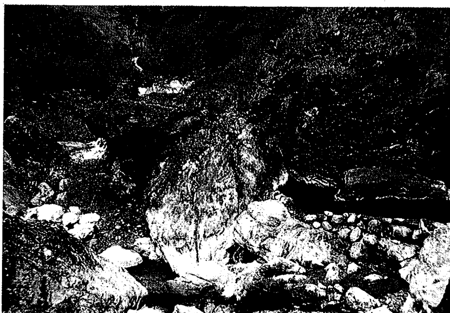
Figure 5.0.3. Mud-mortar masonry diversion used in the dry season to capture all the water in the stream. Water is diverted through a small opening behind the stone to block floods from entering the canal.
