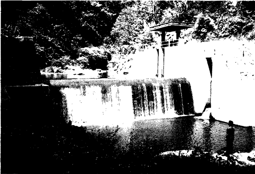
Figure 5.3.5. Reinforced concrete weir that replaced a masonry weir destroyed by a flood, Bali, Indonesia.
