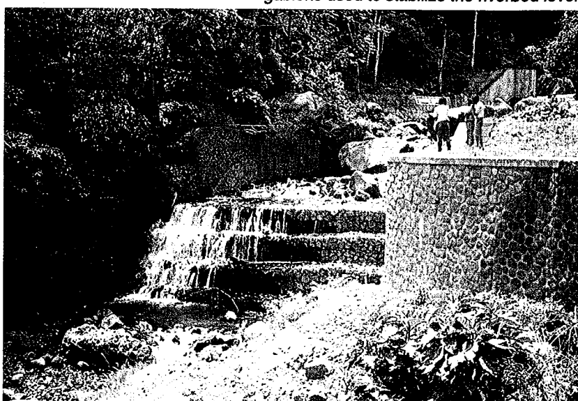
Figure 5.3.2. Close-up view of location where masonry weir failed. Note gabions used to stabilize the riverbed level.
