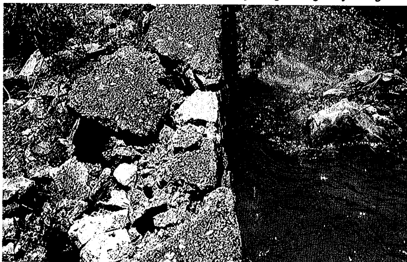
Figure 4.4. Masonry lining damaged by falling rock.
