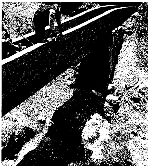
Figure 4.5. Reinforced concrete T-beam aqueduct combining good design and workmanship.
