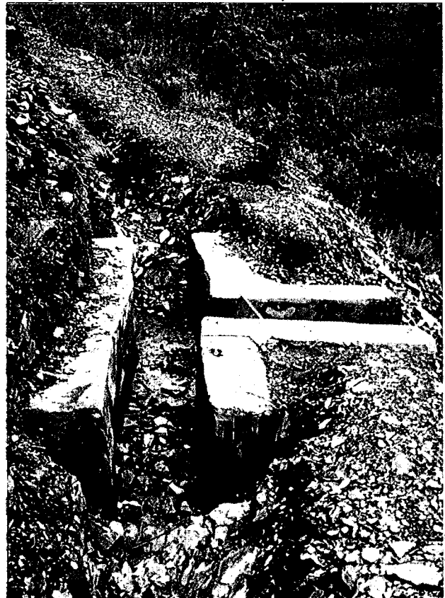
Figure 4.3. Gated rain water escape in remote location.
