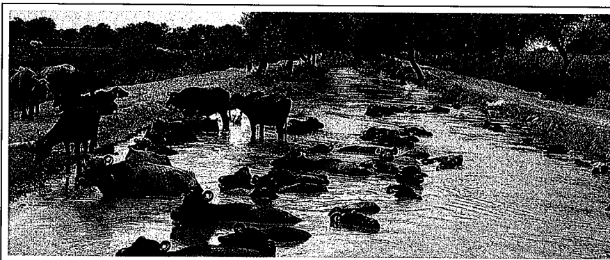
Damage to banks by wallowing buffalo is one of many on-farm factors that eat away at system efficiency and productivity.
