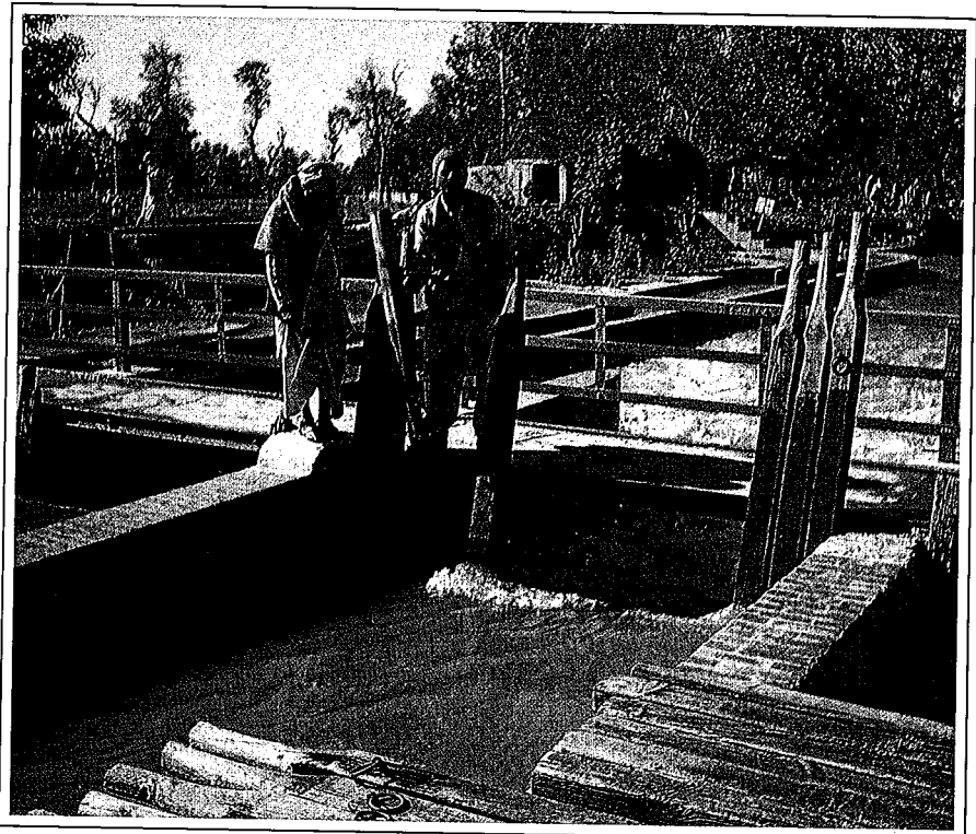
Using wooden billets to augment flow levels – an improvised response to deterioration of elderly control structures in Punjab.
