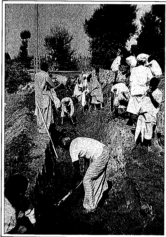
Farmers install a turnout as part of watercourse improvement efforts by a Water Users' Association.
