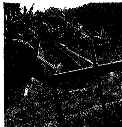
Indonesia is re-evaluating its approach to O&M, like many Asian countries, to stop the deterioration of existing systems.
