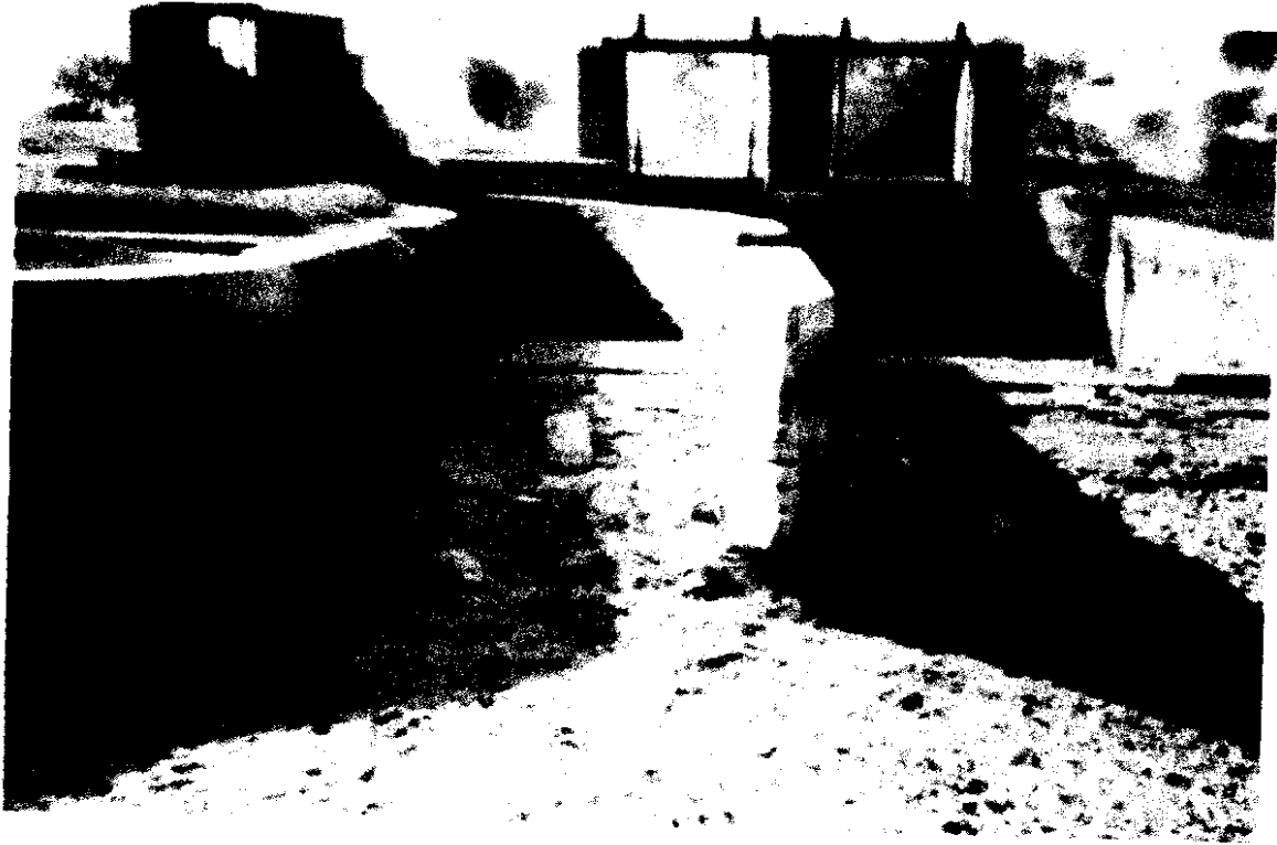
Figure 22. Picture showing gated fall structure (at the right) and the head regulator of Nakewah Minor (at the left) just upstream at RD-63 + 630 of Daulat Distributary.
