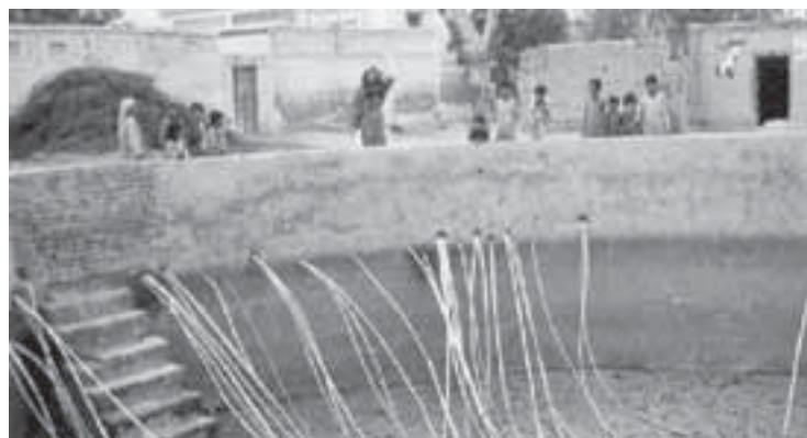
Villagers tapping small community reservoirs ( diggis )—the water is either hand carried or supplied through PVC pipes to the households.
